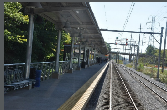
Double Track Platform
